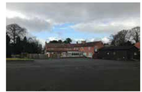
Fig. 8: Rear / South elevation of existing public house.
