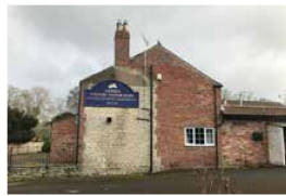
Fig. 6: Gable end (west facing elevation).
