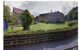
Fig. 11: Rear / east elevation of existing public house.
